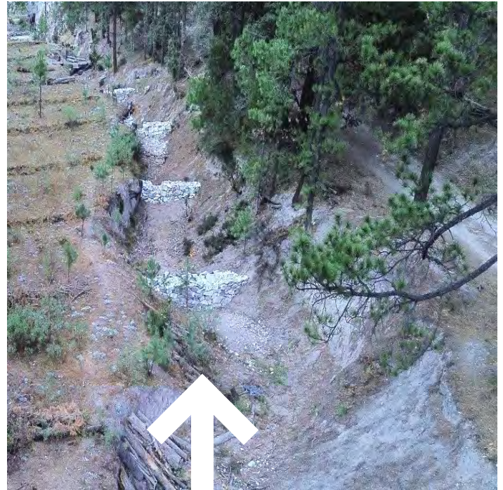
A closer look at a filtration dam in action reveals the effectively trapping of sediment and water, playing a crucial role in preventing erosion and promoting seed germination.
