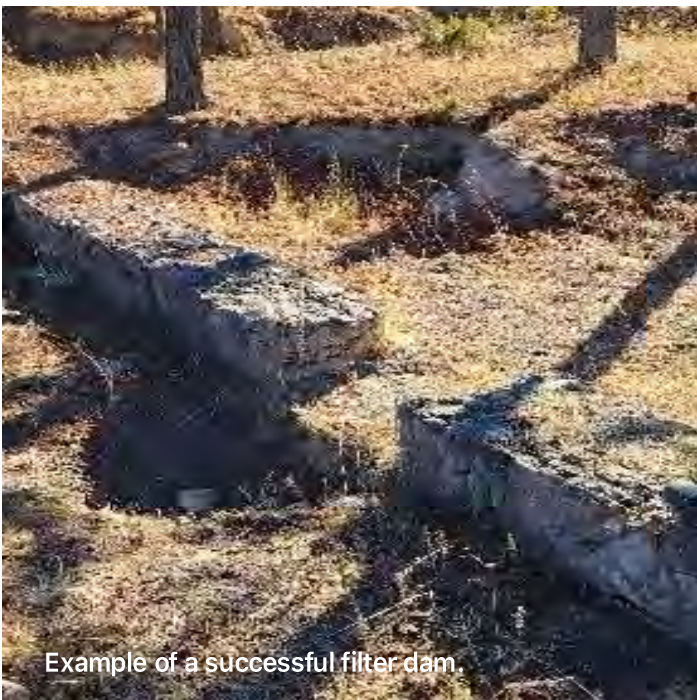
A closer look at a filtration dam in action reveals the effectively trapping of sediment and water, playing a crucial role in preventing erosion and promoting seed germination.
