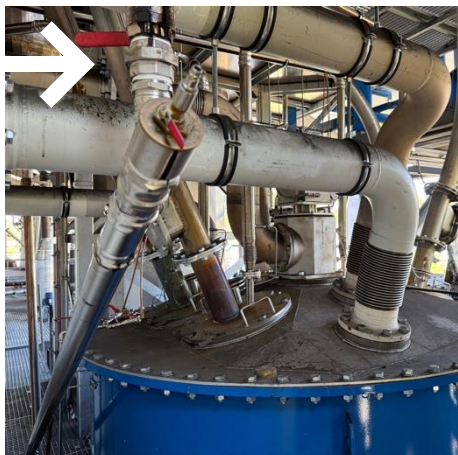
Pipes carry feedstock to the reactor.
