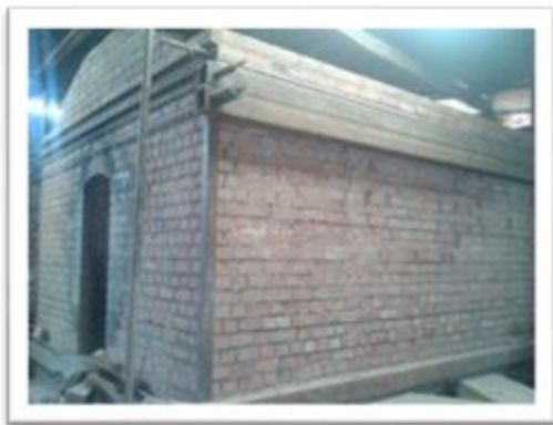
Figure 2: Newly constructed Ugastove kiln
